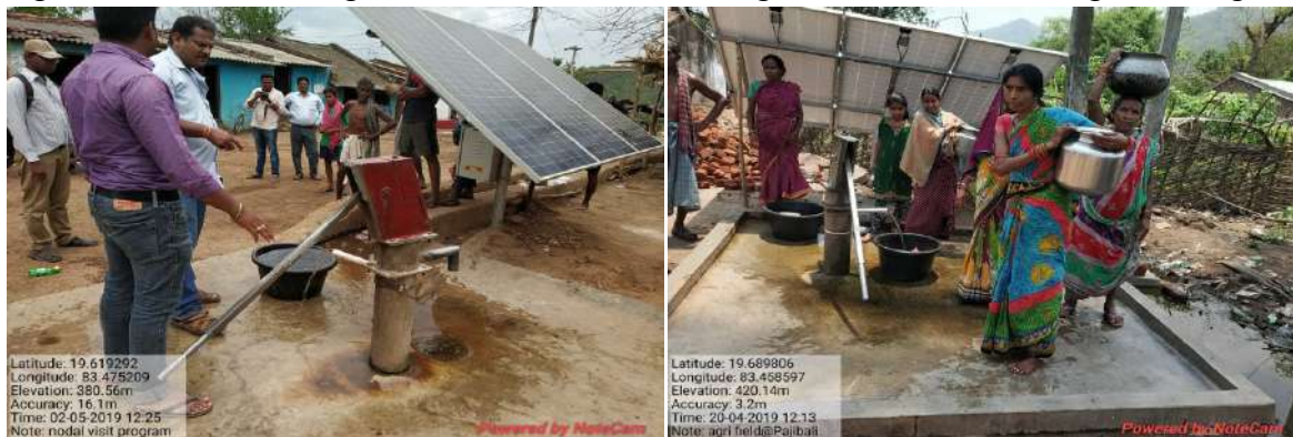
Fig: Solar Drinking water system in connection with tube well
