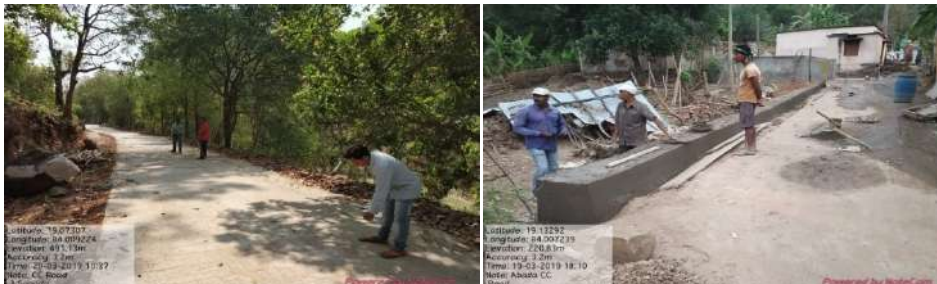
Fig- Const. of CC Road at Sagada to Angara and Const. of CC Road with Side wall
