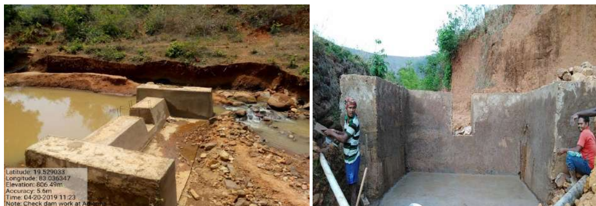
Fig: Check dam works at Adiguna and Kantamal villages during construction
